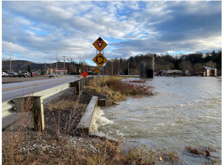
Jeffersonville Flood Bypass Culvert (July 2023)
